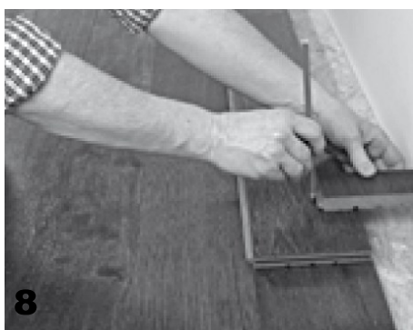
8. When finishing the last row a piece of off cut can be placed over the board to be cut in and used to scribe the shape of the wall.
