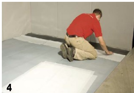
4 FOLD BACK THE PROTECTIVE FOIL OF THE ADHESIVE LAYER OVER A WIDTH OF ONE OR TWO BOARDS, THE ADHESIVE LAYER IS NOW EXPOSED
