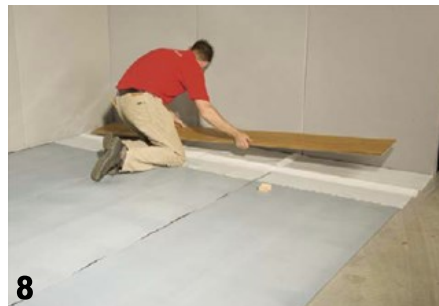
8 THE FIRST PARQUET SECTION OR BOARD IS NOW POSITIONED ON THE SPARE FILM
