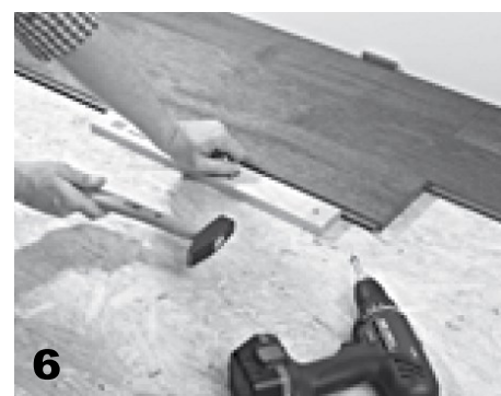
6. with the tapping block from your solid wood / engineered floor fitting kit Join the planks together by tapping gently with a hammer.
