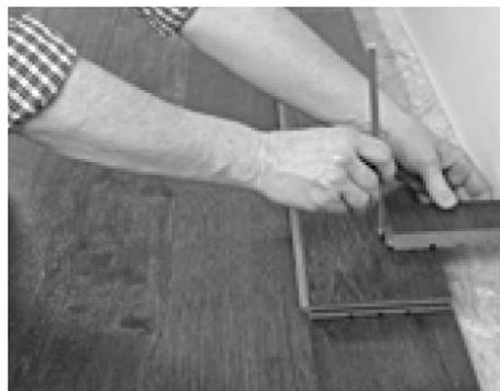
8. When finishing the last row a piece of off cut can be placed over the board to be cut in and used to scribe the shape of the wall.
