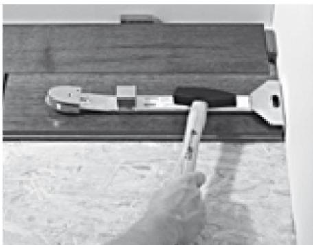
7. A pull bar or pulling iron can be used to help seat the end planks effectively
