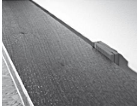
2. An allowance for an expansion gap needs to be maintained by placing wedges at the perimeter edge of the floor. A minimum expansion of 10mm needs to be allowed, for larger rooms this needs to be increased.
