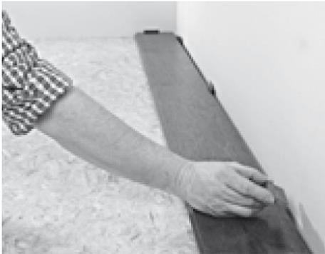
1. Cut the first row to size, centre and align the planking to the area
