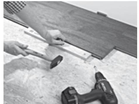
6. with the tapping block from your solid wood / engineered floor fitting kit Join the planks together by tapping gently with a hammer.
