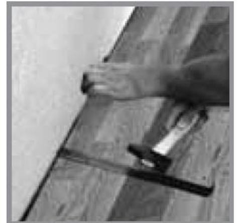
6. The strips for the final row will need cutting to width making sure that the expansion gap is allowed for. The use of a pull bar or joint puller will be needed for this final row, wedges can be removed 24hrs after laying.
