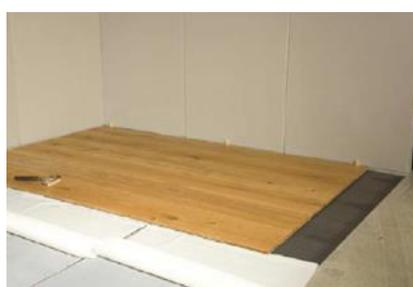
11. From here onwards, several rows can be positioned seamlessly before the protective layer between the wood and the underlay is removed.
