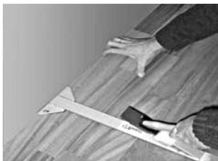
4. The positioning of wedges between the plank and the wall will allow an expansion gap all around the edge of the room, a minimum expansion of 10mm needs to be allowed, for larger rooms this needs to be increased, continue to lay your floor checking regularly for alignment and squaring if required.
