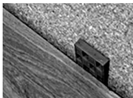
6. Fitting the final row will require the use of a pull bar or pulling iron this specialized tool makes up part of the solid wood / engineered fitting kit along with wedges and a tapping block. The wedges placed around the edge of the floor to maintain the expansion gap can be removed after 24hrs.
