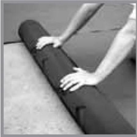
1. Lay out an underlay suitable for the sub floor, a vapour barrier will be required for Concrete or stone based floors, if using Fibre board a 2mm expansion gap between boards will be required
