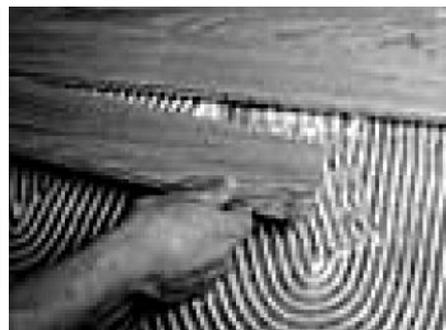
3. Set the plank into the adhesive, pressing it in making sure of a good contact and subsequent planks in a random A symmetric pattern and allowing for an expansion gap at the edge, this type of installation does not require you to glue the tongue and groove.
