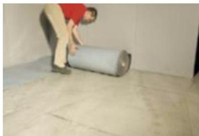
1. Roll out the underlay over the polythene moisture barrier in rows next to one another (the underlay strips must not overlap)
