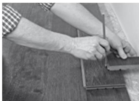
8. When finishing the last row a piece of off cut can be placed over the board to be cut in and used to scribe the shape of the wall.
