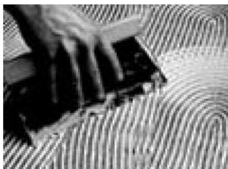
2. With a 6mm wood floor adhesive trowel the flooring adhesive is spread in a criss-cross pattern onto the sub floor as seen in the picture its advised to work on small areas at a time. Your wood floor adhesive will yield about 1m<sup>2</sup> of coverage to 1000g of adhesive.
