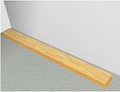
1. Start in a left hand corner of the room with the locking strip (groove) facing the room. A minimum expansion of 10mm needs to be allowed, for larger rooms this needs to be increased.
