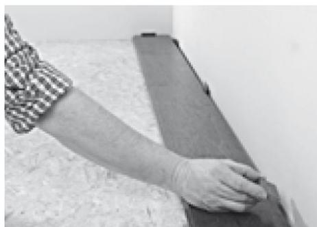
1. Cut the first row to size, centre and align the planking to the area
