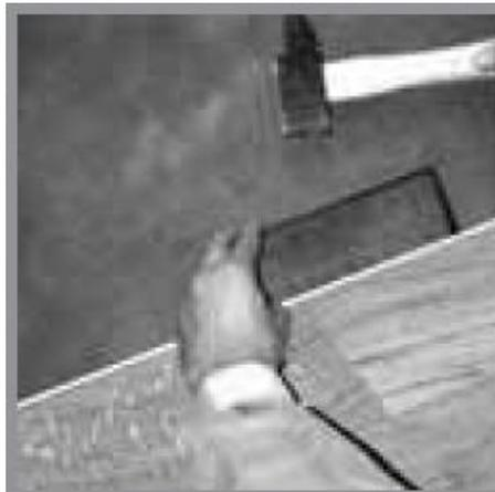
5. A tapping block will avoid any damage to the tongue while the strips are being fitted together
