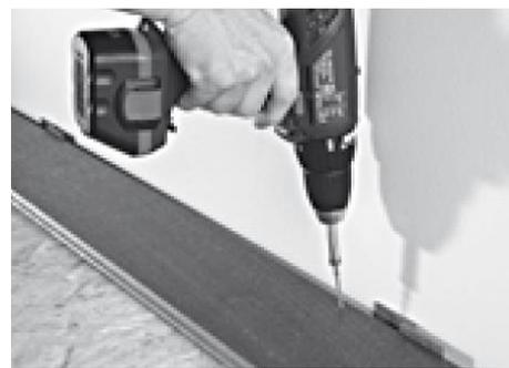
3. The planks in the first and last rows are fixed from the top with either nail or screw, the fixing is placed around 15mm from the edge of the plank
