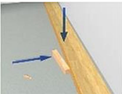
7. When the whole row is completed, remove the wedge and press the boards down, position the floorboard by tapping with a block of wood.
