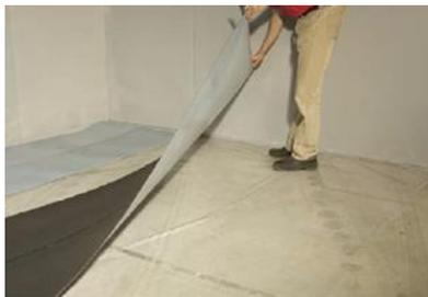
2. Turn over the underlay so that the smooth protective layer is on the upper side.
