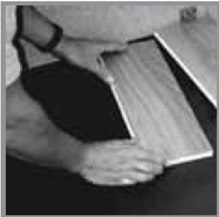
4. When starting the second row use the off cut salvaged from the end board of the first row making sure this is at least twice the width of the strip itself. Clean off any glue traces that may have squeezed out during fitting immediately.
