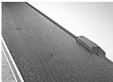
2. An allowance for an expansion gap needs to be maintained by placing wedges at the perimeter edge of the floor. A minimum expansion of 10mm needs to be allowed, for larger rooms this needs to be increased.
