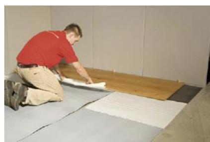
10. The second board is tapped into the first to give a tight fit, following this, the spare film between the underlay and the boards is removed. From now on work is carried out with the actual protective layer of underlay.
