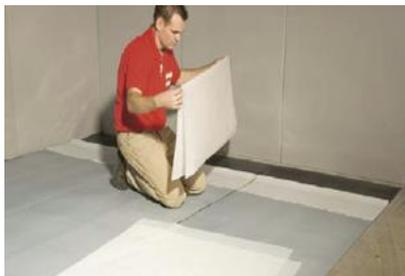
5. Fold a piece of film taken from some spare underlay in two, don't worry keep it safe and the underlay can be used later.
