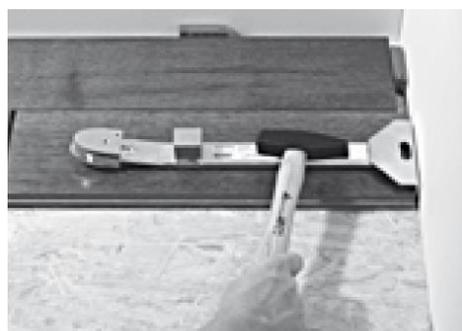
7. A pull bar or pulling iron can be used to help seat the end planks effectively
