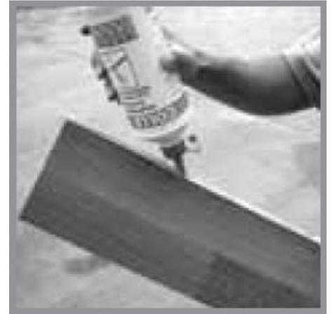
3. Apply glue to the upper edge of the tongue to the end or head joints as well as along the length of the first row.
