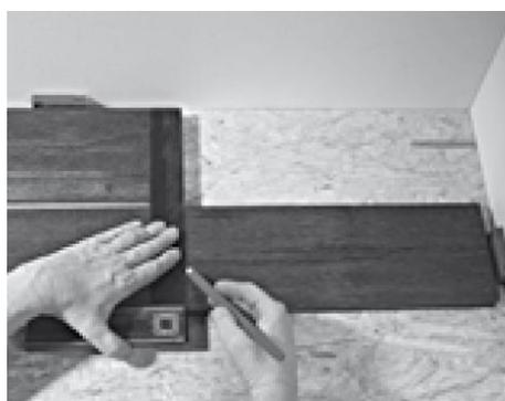
5. The row finishes by cutting your plank allowing for the expansion gap the cut off piece will return and start the second row
