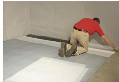
6. Carefully place the spare film onto the exposed adhesive layer with the fold facing the wall.
