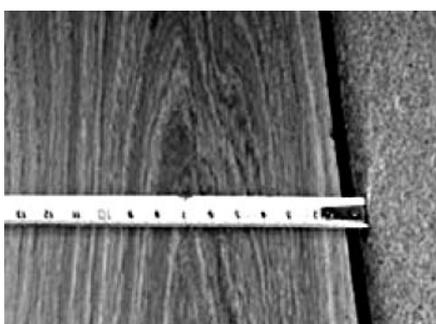
5. the last row of planks to be fitted will need to be tailor cut to suit the width left less the expansion gap. As part of preparation if the width of the room is measured and it leaves the final row to be less than 50mm reduce the front row to make it the same as the last.
