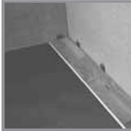
2. The first strip of wood is placed with the groove edge towards the wall, making sure that the wedges are placed between the strip and the wall. A minimum expansion of 10mm needs to be allowed, for larger rooms this needs to be increased.
