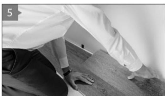
5. The second plank of row one will also be a full size long plank, once again angle the long side of this plank into the long side of row two's first plank, slide the third plank to the left so the short end meets the short end of the first plank of row one, it is then lowered to lock into position.
