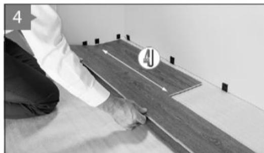
4. The first plank of row two will be a full size plank, angle the long side of row two's first plank onto the long side of plank one of row one, lower plank one of row two to lock them both together making sure there are no gaps.
