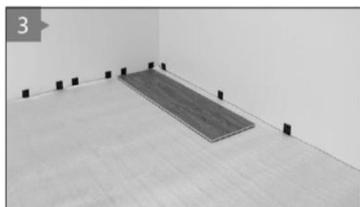
3. It is of the utmost importance that the first row is installed straightly to achieve this both rows one and two will be installed together alternating between planks at each stage, this will only need to be done for the first two rows. Row one is started with a cut down half plank.
