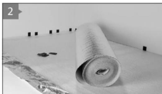
2. The use of a suitable LVT underlay not exceeding 1.5mm is recommended assisting with the installation and slight unevenness in the subfloor. To maintain an even expansion gap place spacers to give an equal distance between the wall and the plank.
