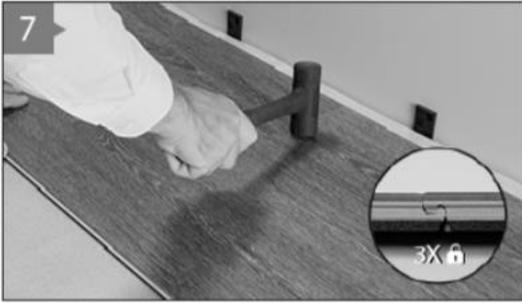
7. The use of a rubber mallet in conjunction with a tapping block can be used to fully secure the locking system. This requires no more than a tapping force.
