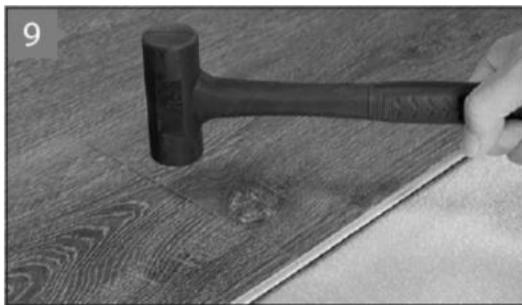
9. Continue to use the rubber mallet and tapping block to fully secure the locking system. Remember this requires no more than a tapping force.
